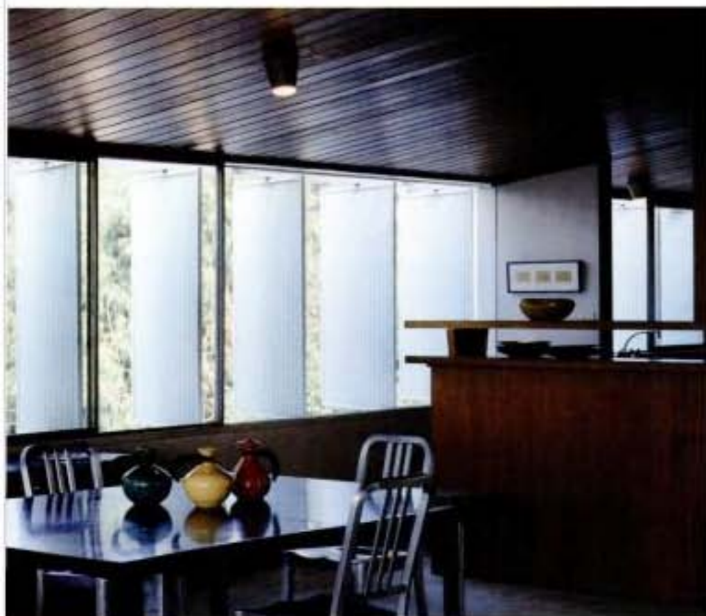
(left) Perforated steel louvers were installed to provide protection from the east and west sun without interrupting the views. During the renovation, Lautner determined that these were still the best way to provide shade from the harsh rays, since the lot did not have room for additional trees. The lack of acreage on the lot is perhaps Rodman and Friedberg's one regret about the house. (above) Lautner's original Douglas fir kitchen countertops still remain—as sturdy as the day they were installed.
